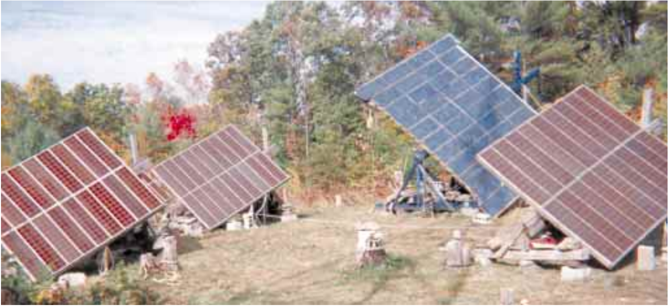
Four of the five PV arrays. Total PV output is about 3,000 watts.
