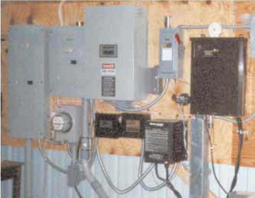
Bill's two systems converge, but remain discrete, on the power wall in his shop.
