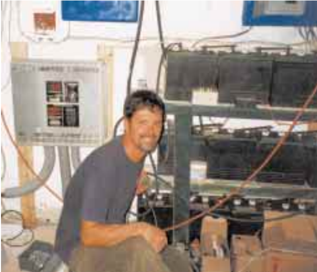
Lonnie Gamble in his battery room, with the Whisper controller visible in the left rear.
