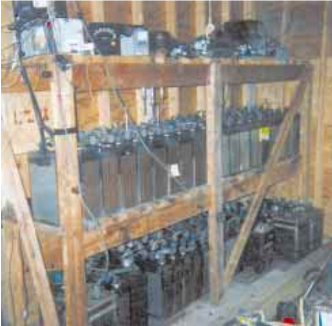
Half of the 120 lead-calcium cells.
