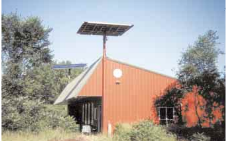
Bill's shop, with two Wattsun dual-axis trackers which hold thirty-four Solarex MSX-64 PV panels for two independent systems.
