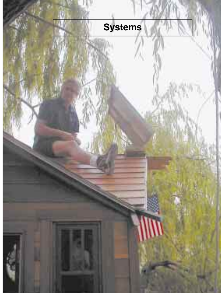
Up the tree, on the roof, with the PV.
