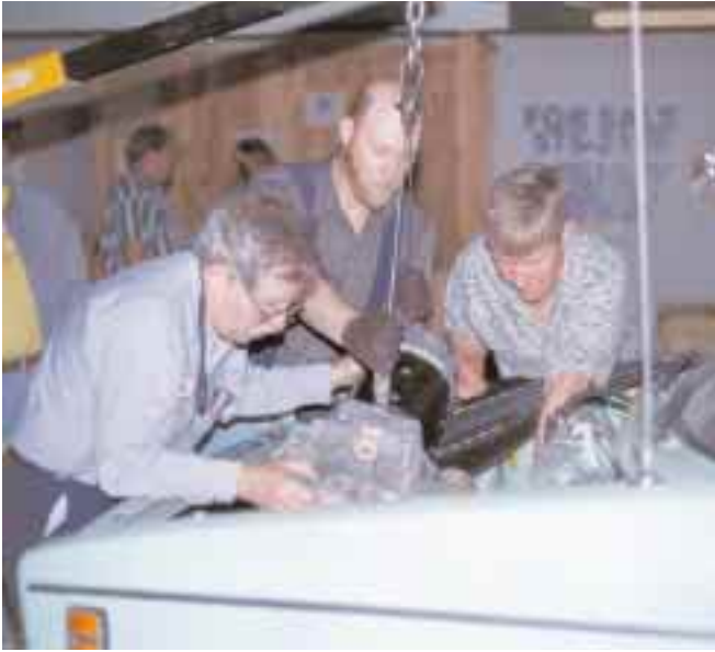
Lowering the new electric motor into place.
