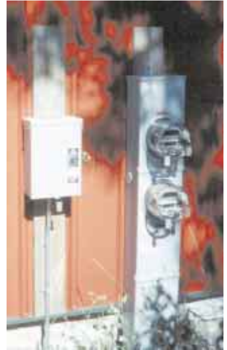
Safety lockout and two KWH meters for the intertie system.
