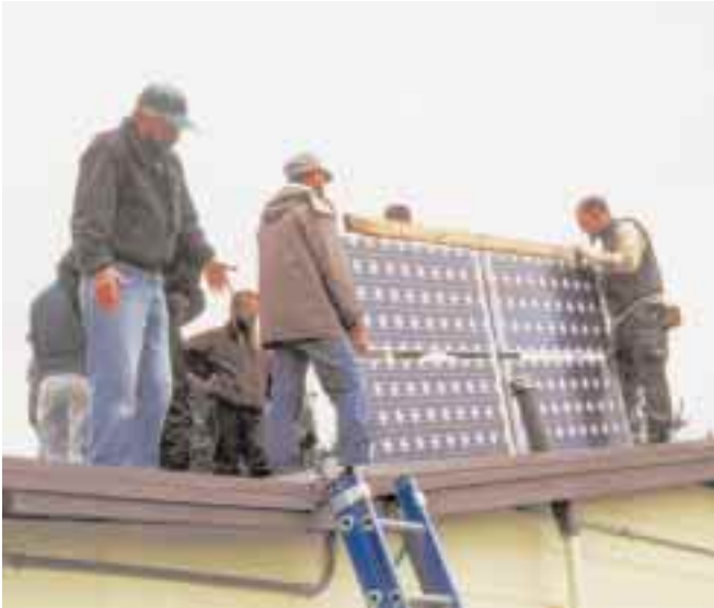
The fun part—puttin' panels on the roof.
