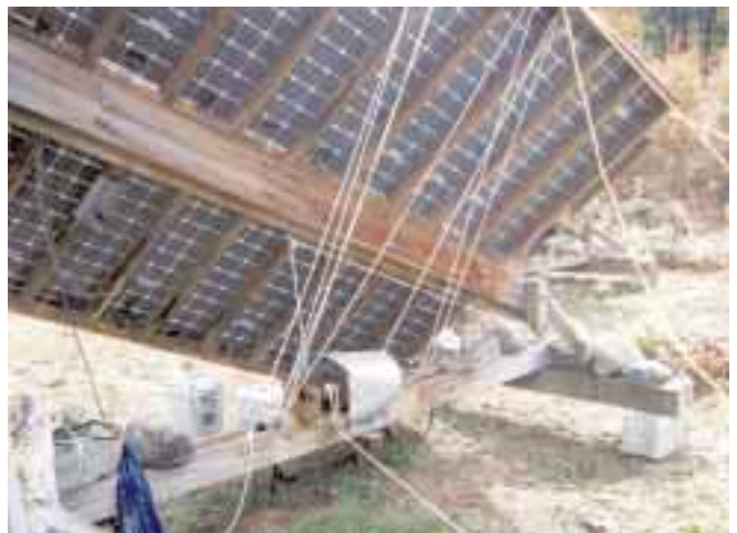
Nylon ropes from winch motors provide 8 seconds of tracking correction once every 15 minutes.
